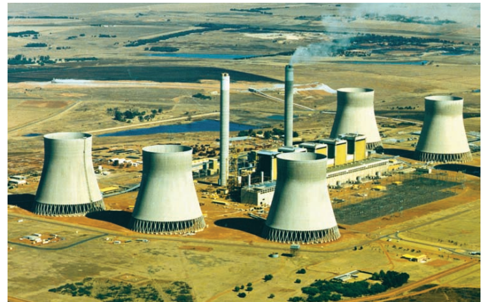
Indirect Dry Cooling —An indirect dry natural draft condensing system, in the example above, couples a dry cooling tower with a steam surface condenser. Such a condensing system is particularly suited for large power plants. The concept can also be applied with mechanical draft dry towers over a wide range of plant sizes.
